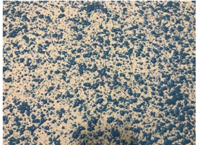
FIG 1. CORRECT COVERAGE – SPLATTER APPLICATION
