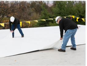
WeatherBond's Peel & Stick (PAS) TPO roofing membrane with pre-applied adhesive combines the energy efficiency and durability you expect from WeatherBond's TPO with the easiest installation in the industry. Our peel and stick technology saves labor and improves membrane performance, which translates into satisfied building owners.
