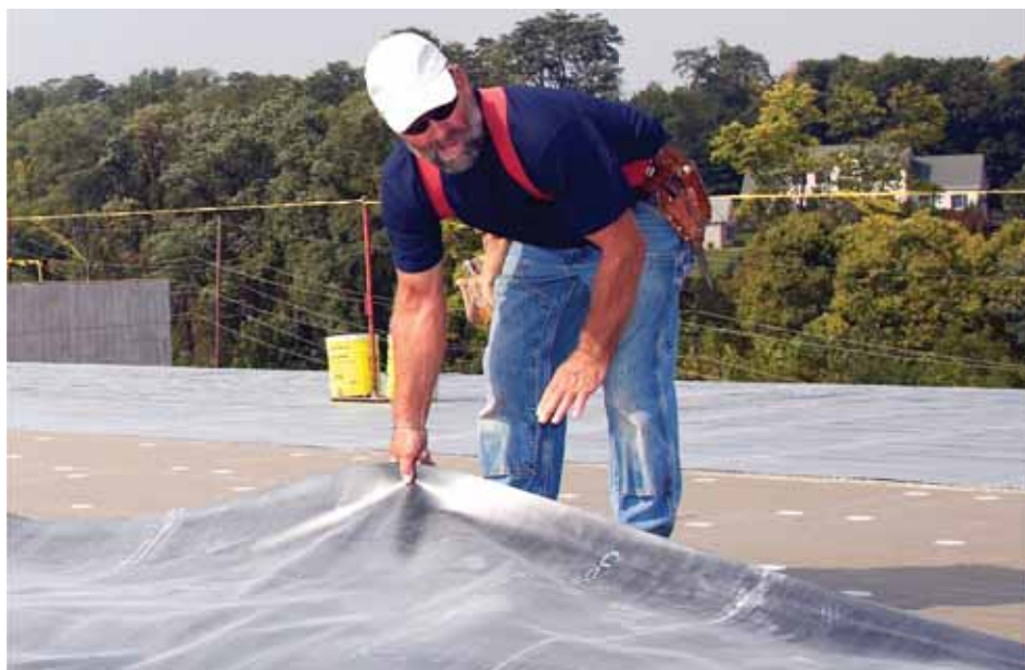
WeatherBond EPDM with Pre-Applied Seam Tape formats for wide-width sheeting includes a single-fold sheet.
