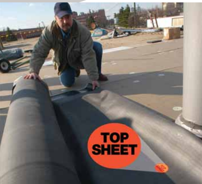
Locate the orange "TOP SHEET" sticker on 2-packs to ensure proper roll-out.
