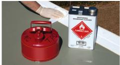
Clean the surface to be painted using WeatherBond's Weathered Membrane Cleaner and allow to dry thoroughly.
