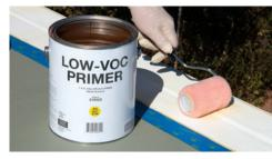
Coat the surface of the product with WeatherBond's standard or Low-VOC TPO Primer.
