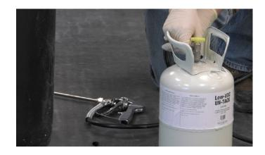
When removing the spray tip of the gun for cleaning or replacement, it is not necessary to relieve the pressure in the gun and hose assembly. Make sure the safety stop on the trigger is positioned to not allow the gun to operate. Wear safety glasses during this procedure and anytime while spraying adhesive.
