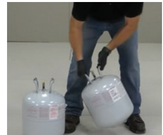
Shaking of A-side and B-side tanks
