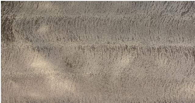
Proper Coverage on Membrane
