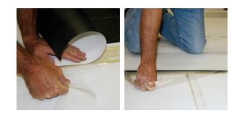
The Weld-Free TPO System from WeatherBond is an energy-efficient, cool roofing option that can be fully adhered or mechanically attached without the use of a heat welder.
